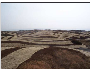
Geojute spread across the moors
